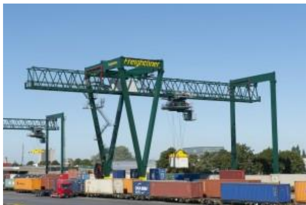
Kuva 49. Freightliner terminaali Southamptonissa ( https://www.freightliner.co.uk/location/southampton-maritime/ )
